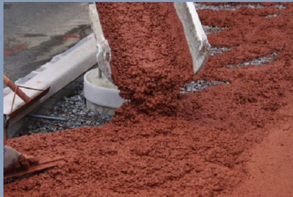
Integral colored concrete
